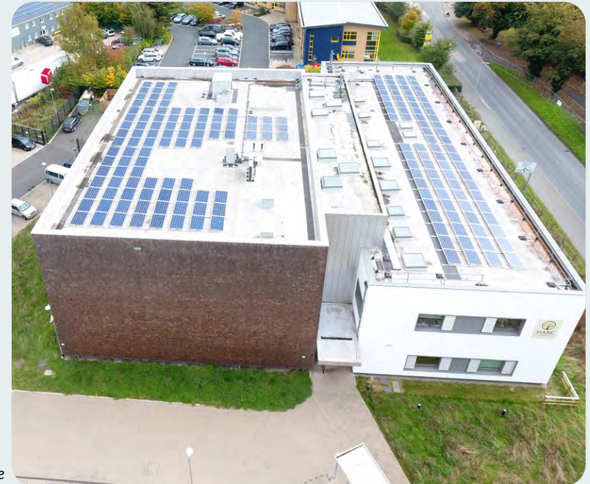
Solar panels on the roof of the Herefordshire Archive and Records Centre
